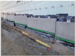
Figure 6 – Pre-cast concrete panels installed throughout the NCC at ground level.
