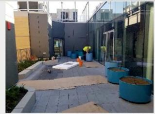
Figure 4 – Pedestal and Paver system installed within the Library's reading garden. Planters being placed with soil.
