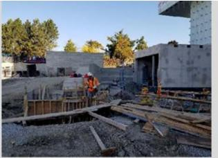
Figure 7 – Formwork being placed adjacent the NCC Maintenance Garage for cast-in-place concrete steps.
