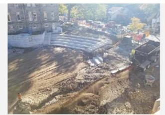
Figure 2 – Donofrio backfilling the now repaired sanitary line within the square.
