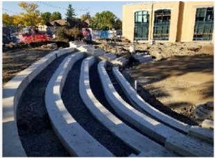
Figure 1 – Amphitheater seating poured and stripped within the square.
