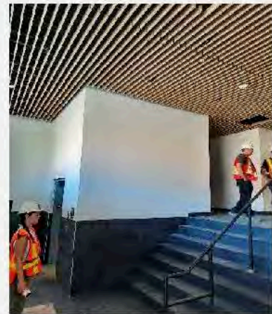
Figure 8 – Main entrance lobby tiling and ceiling is complete. Stainless steel railings to be installed today.
