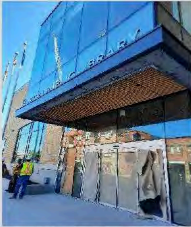
Figure 3 – West entrance canopy not yet completed
