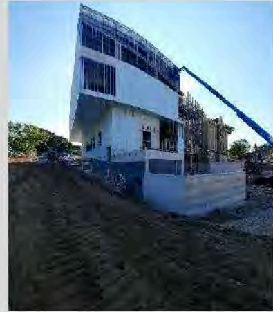
Figure 4 – View of the NCC from the north
