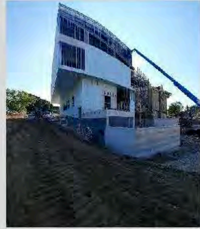
Figure 4 – View of the NCC from the north
