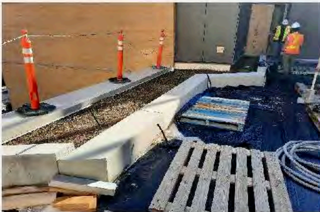
Figure 5 – Reading garden precast planter walls in place. Insulation needs to be levelled
