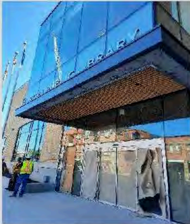
Figure 3 – West entrance canopy not yet completed
