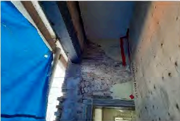
Figure 11 - Masonry work and lintel between the NCC and the school house
