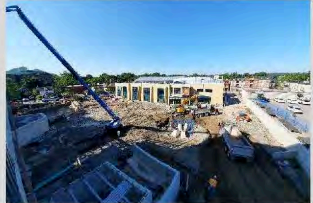
Figure 10 – View over the square from the 2 nd floor of the NCC
