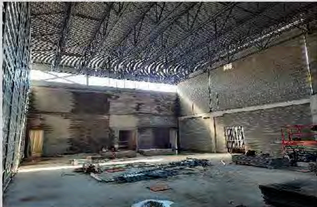
Figure 9 – View of the NCC theatre from the back of the room. Ceiling in place
