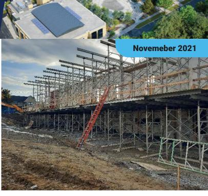
Figure 2: Ground Floor north wall of new Cultural Centre has been poured and stripped
