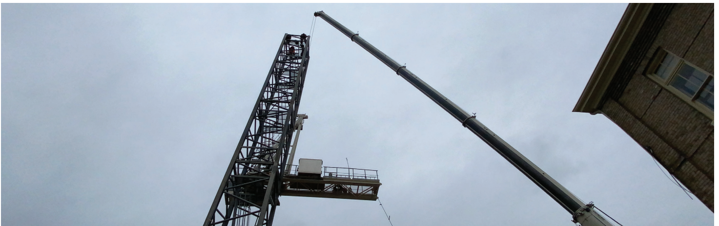
Figure 2: Tower crane installation.
