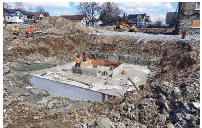
Figure 6: Tower crane pad has been poured.
