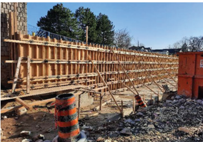
Figure 5: Forming for retaining wall at north end being finalized.
