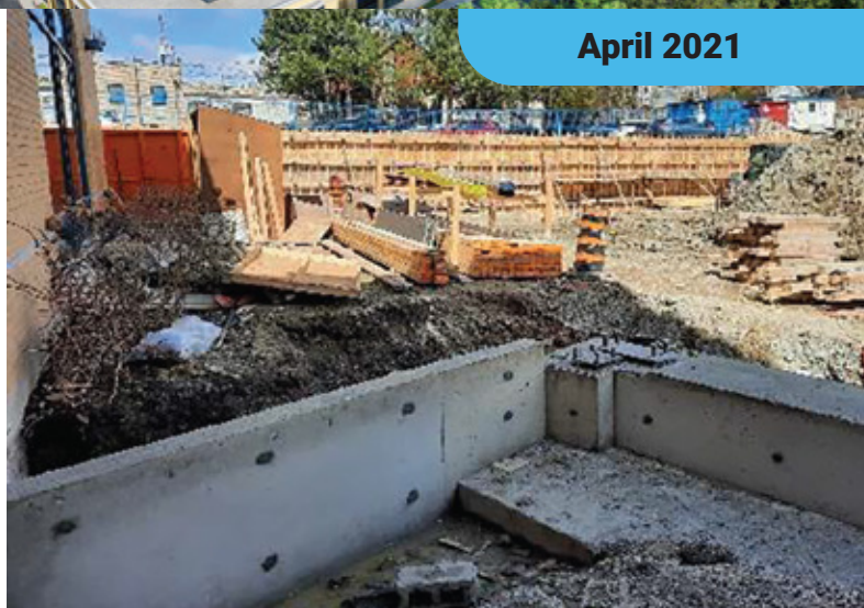
Figure 2: Foundations for bridge poured at east library entrance.
