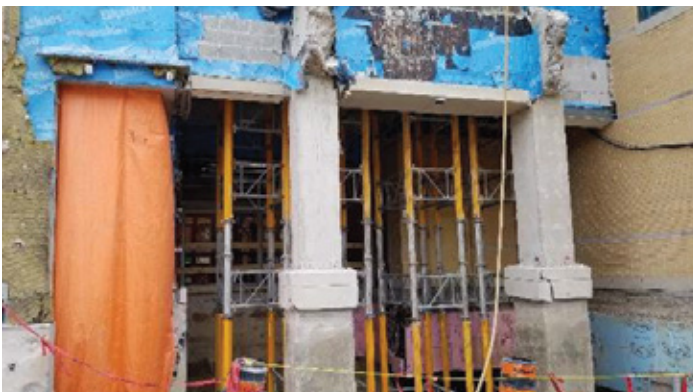
Figure 3: Shoring installed at the west Library entrance.
