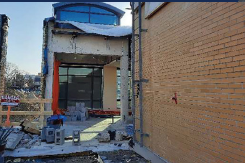
Figure 1: Opening for bridge access has been cut.
